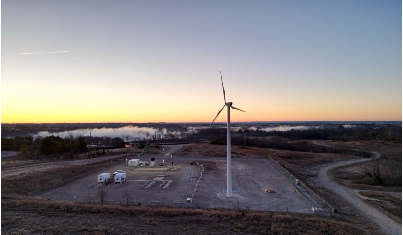
Photo of Kentucky's first utility wind turbine installed in February 2024 at Kentucky Utilities' Renewable Integration Research Facility
